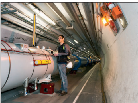
Nedo products in use at CERN
